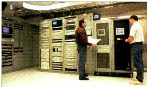
Cartoon Network Brazil is exploring the limits of computers and networking technology. This operation employs traditional 10BaseT networks and FDDI fiber, moving video packets according to commands sent over the slower network. Photo by Mark Hill, TBS, Inc.
