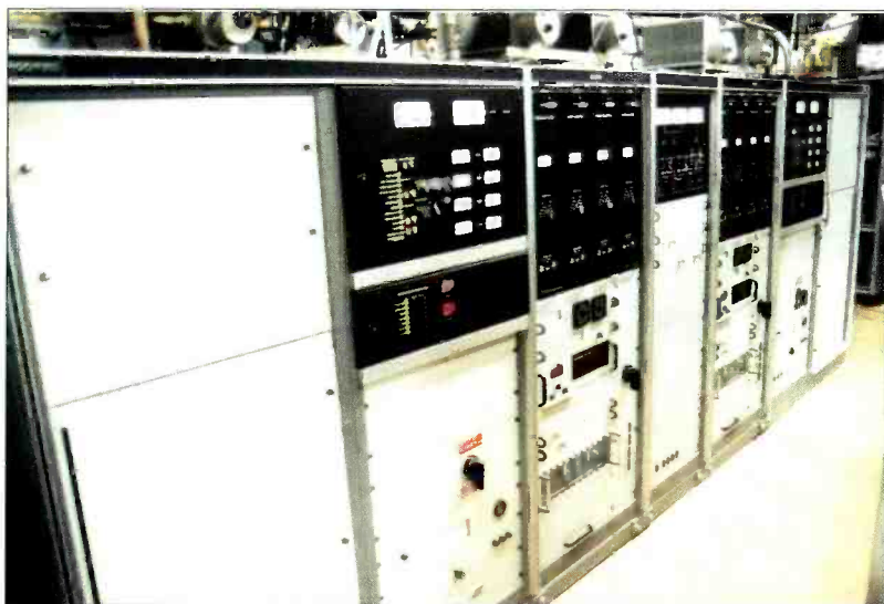
CTN's new Acrodyne transmitter, the Au120D dual-tube 60kW Diacrode transmitter with 120kW output.
