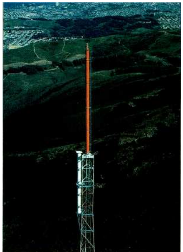
Andrew Corporation's TRASAR broadcast antennas can be engineered to be suitable for NTSC and DTV transmission.
